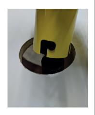
3. Cut the ABS or PVC 1 ½" pipe 3" shorter than the distance between the floor and the P-trap.
