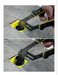
**13.** Apply provided lubricant halfway up the tailpiece and position the bathtub and tailpiece in line with the Drop-In Drain.
