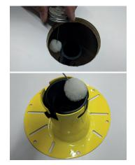
2. Measure the distance from the inside of the P-trap to the top of the floor.
