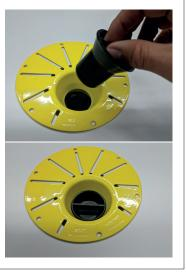
8. Secure the Drop-In Drain to the subfloor with screws or cement.
